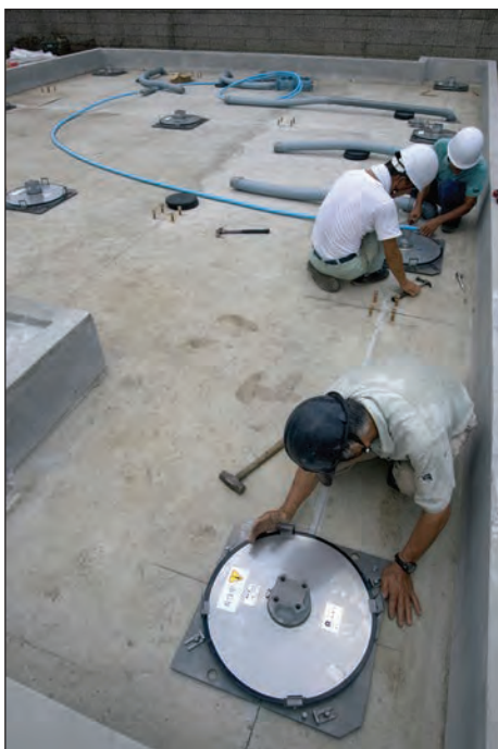
Workers install ball bearing slides to earthquake-proof a house
